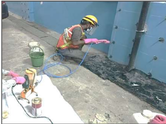
Epoxy Grouting
