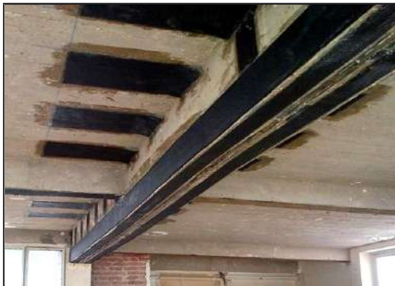
Fiber Wrapping/ laminate
