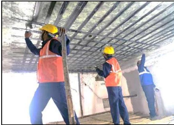
Fiber Wrapping/ laminate
