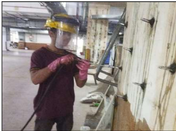
Epoxy Grouting
