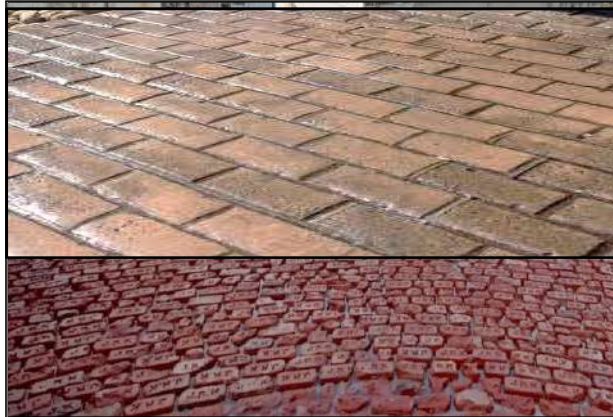
Brickbat coba with Stamped Concrete
