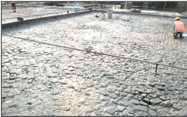
Acrylic coating on brick bats/slab
