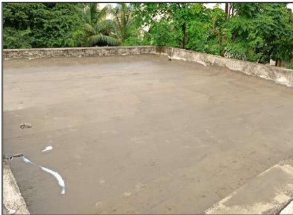
Acrylic coating on brick bats/slab
