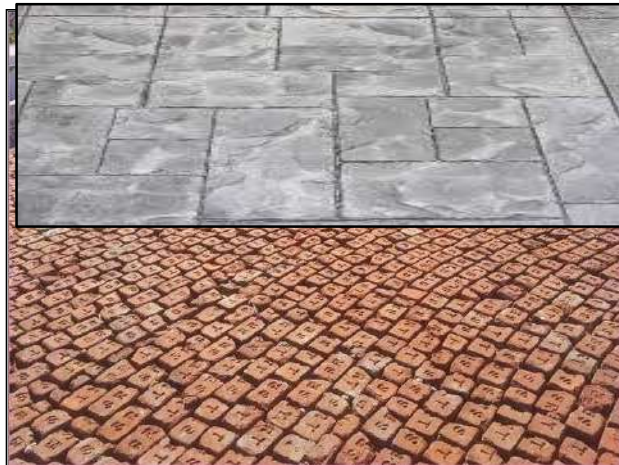
Brickbat coba with Stamped Concrete
